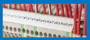
Industry 4.0 is leading to increasingly complex connection technology and a correspondingly high demand for systematic and fast identification inside the control cabinet.
